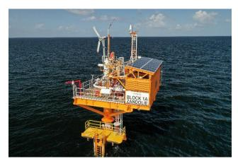
Zandolie is a single well, conductor-supported platform with a nameplate capacity of 40 MMSCFD. The field development builds off the existing Iguana Infrastructure enabling a more compact topside structure that is lighter and more efficient. The space saving achieved also minimises the use of steel in the design allowing for a modular design and greater use of local fabrication services.
